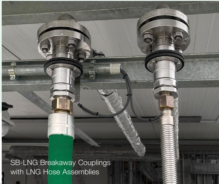
SB-LNG Breakaway Couplings with LNG Hose Assemblies
